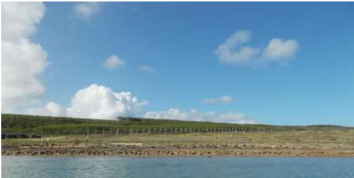
Figure 175: rocky coast in the west backfilled area
